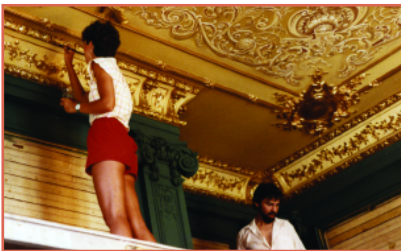
Cornice molding enhanced with the application of gold leaf.
