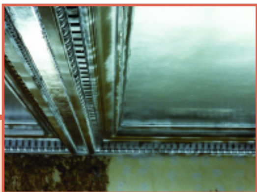
Ceiling after application of aluminum leaf while awaiting glaze.
