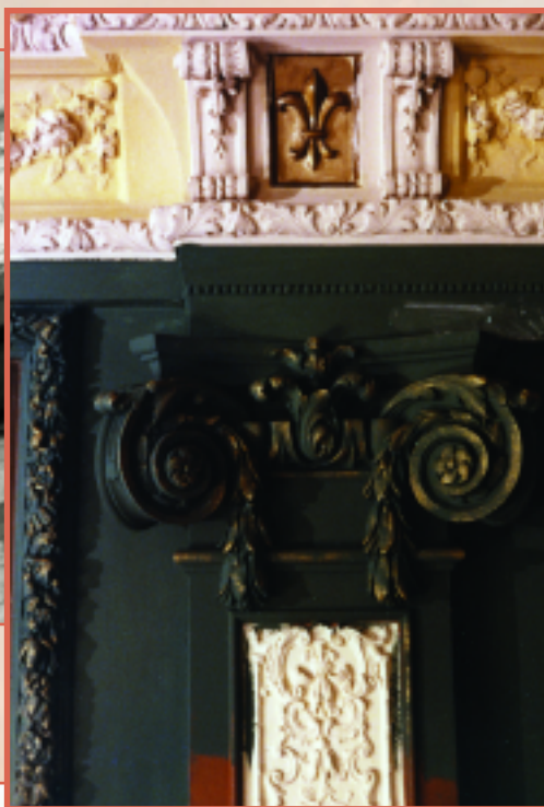
A pilaster is primed and historic paint is added.
