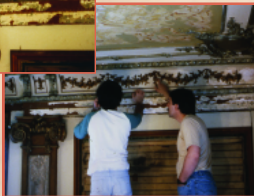
Conservators assess conditions of architectural elements.
