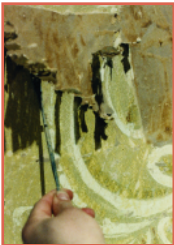
Paint is carefully removed to reveal foliate mural surround.
