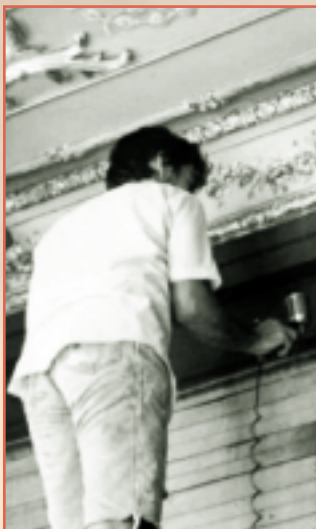
Conservator applies a historically-accurate green paint to wall surfaces and architectural elements.
