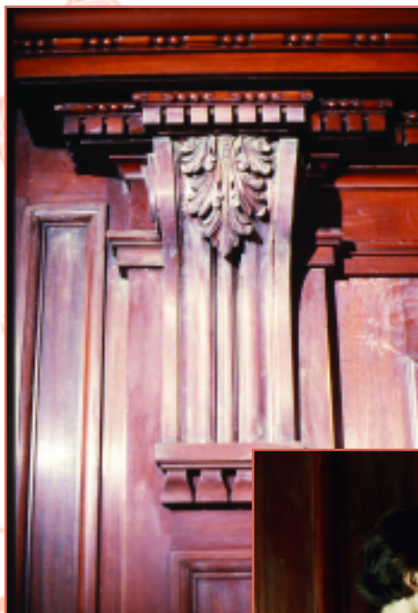
Mahogany woodwork door entablature and corbel undergoing restoration.
