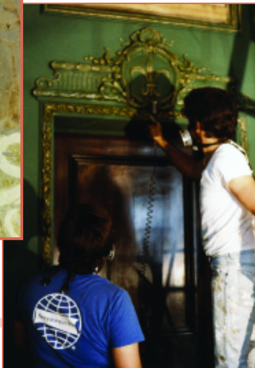
Conservators apply bronze powder to architectural elements using an airbrush.
